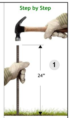
Use hammer to drive rebar into ground. Leave approximately 24" above ground.
